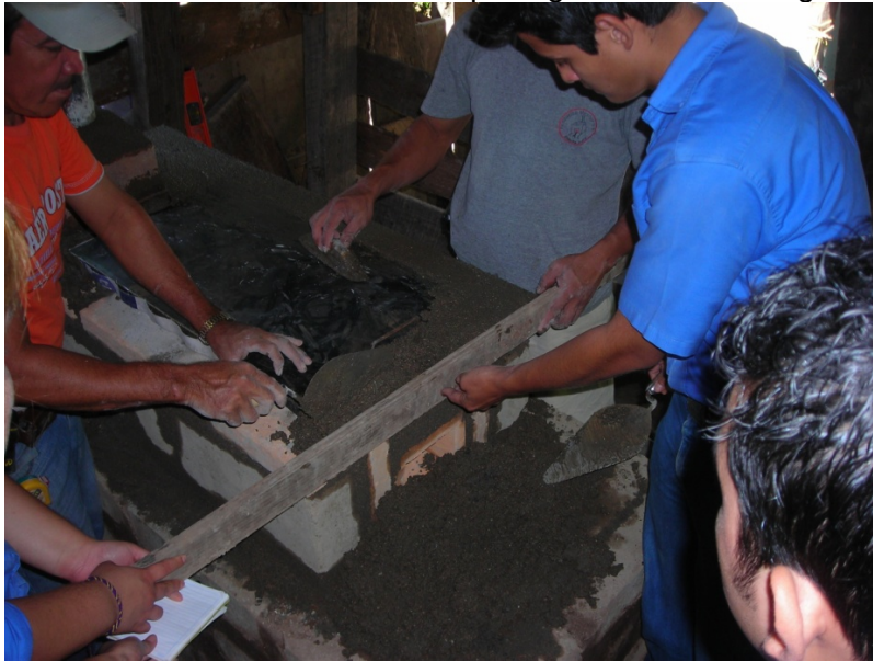
Photo 7: Zamorano students assisting technicians from the Proyecto Mirador in the installation of a Justa 2X3 stove in the house of Doña Delfa Lagos.
